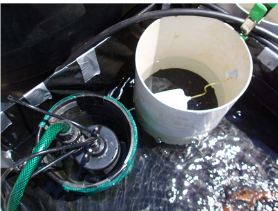
Fig. 3. Submersible pump in well, and float-shutoff for water height control before adding Perlite.
